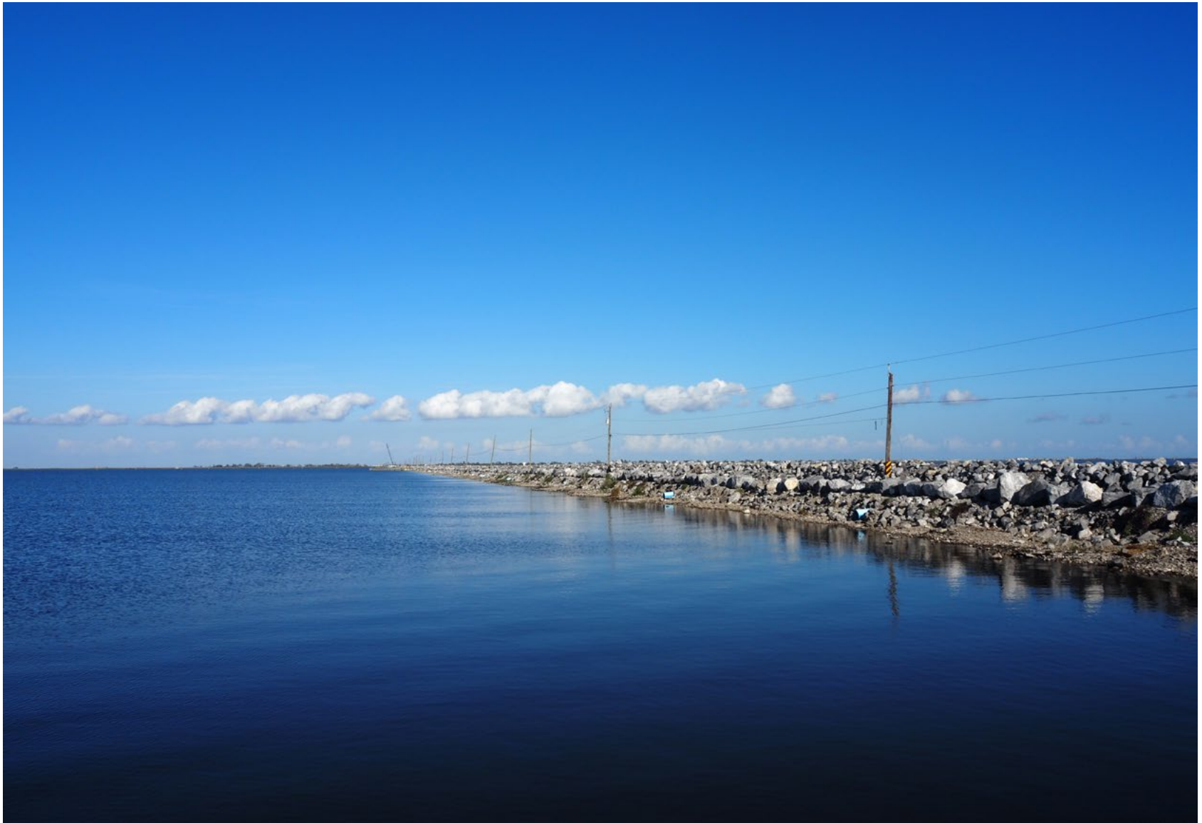
View from a Pier Island Road, Terrebonne Parish
