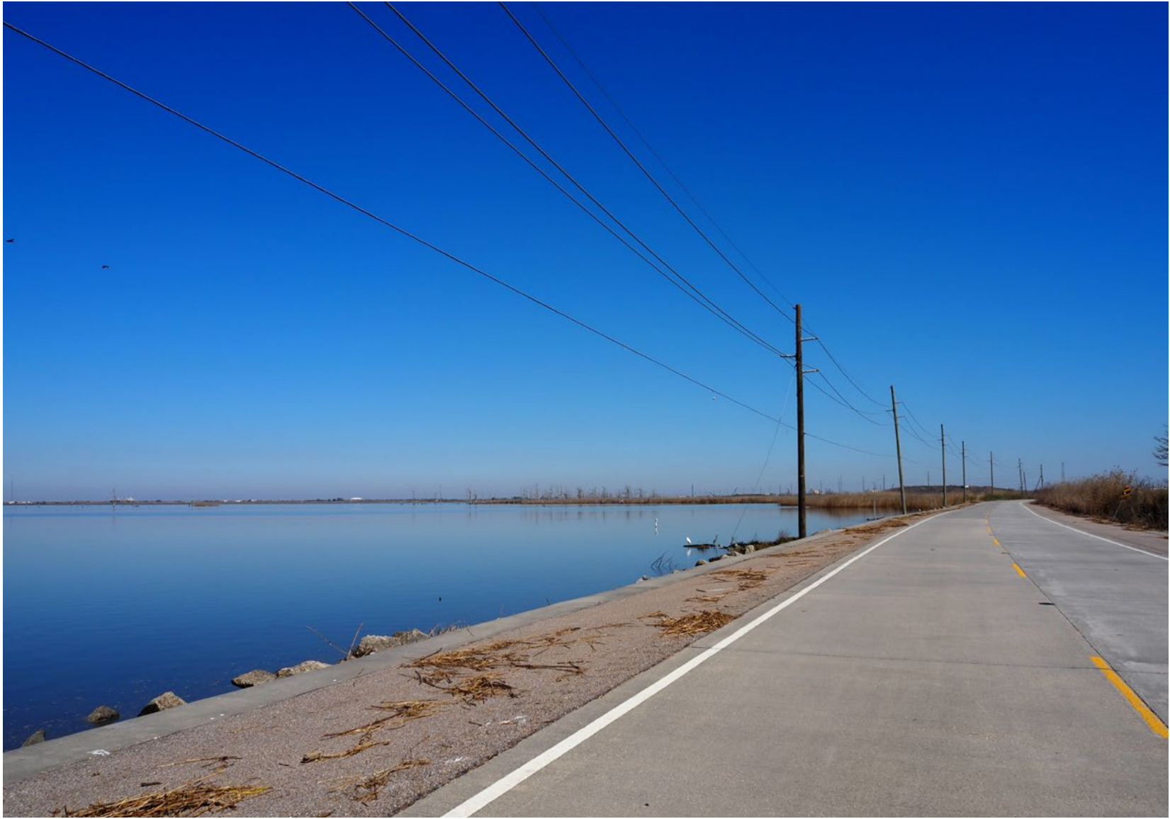
Poles along LA-23, Venice, Plaquemines Parish
