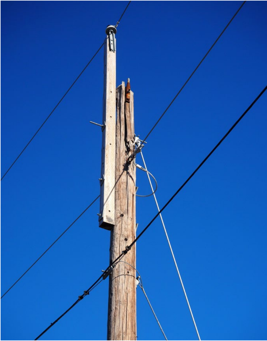
Pole repair Island Road, Terrebonne Parish
