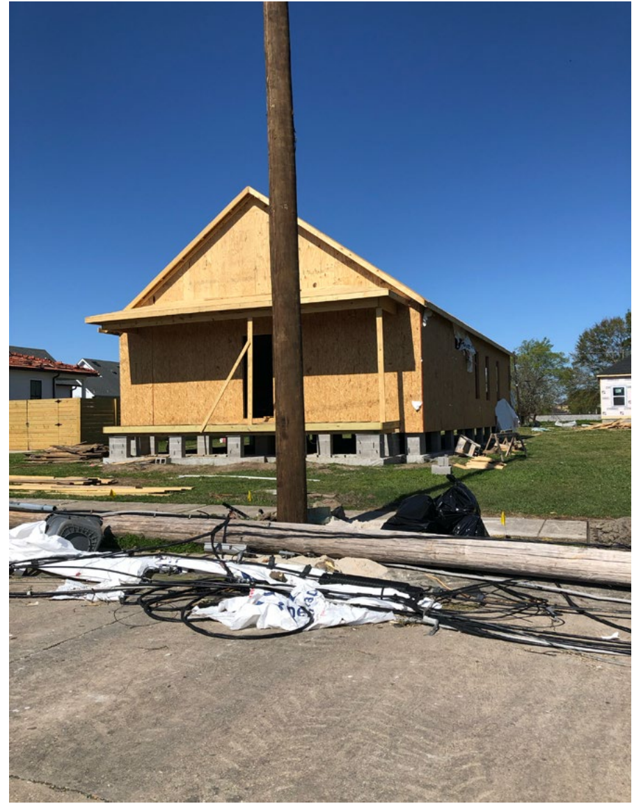
Pole being replaced after tornado Arabi, St. Bernard Parish
